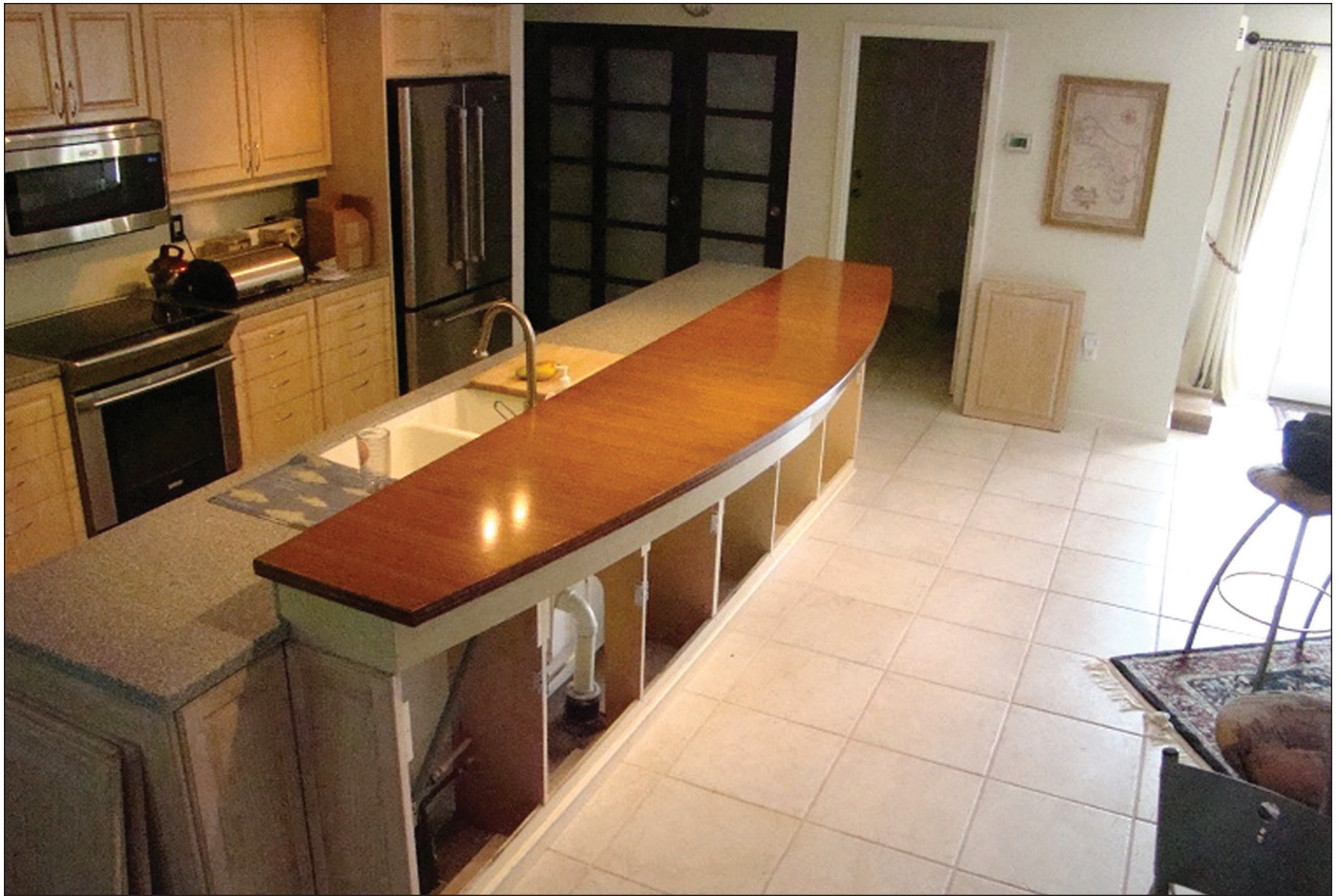
Bamboo, as used in this counter top, is a green alternative to the ever-dwindling supply of hardwoods. COURTESY PHOTO
